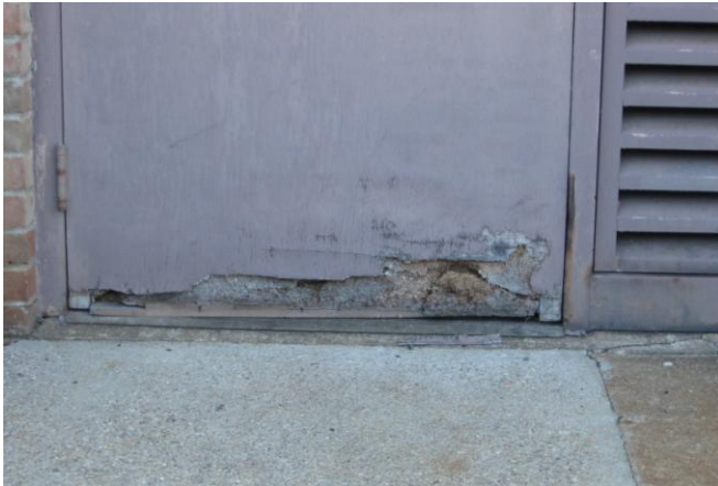
ADM Building – Boiler Room Door
